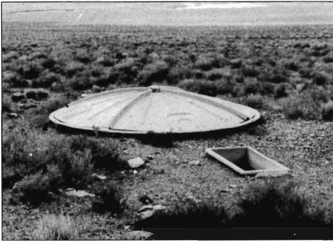
Figure 6. Because of their limited surface area, fiberglass catchments that collect water directly from curved lids are of limited use in areas with insufficient annual rainfall to fill the storage tanks.
