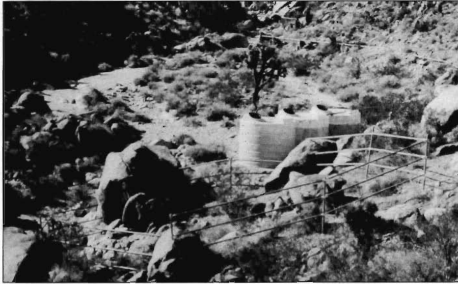
Figure 4. Eight artificial catchments designed to provide a permanent water source for large, native herbivores have been constructed in Inyo County. These catchments capture rainfall from large, natural drainages and store it for use during the hot summer months.
