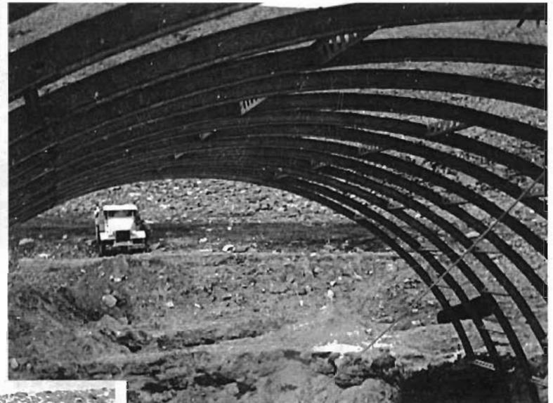
*(Right)* Tom Hanson surveys largely completed rib structure, before plates are attached.
